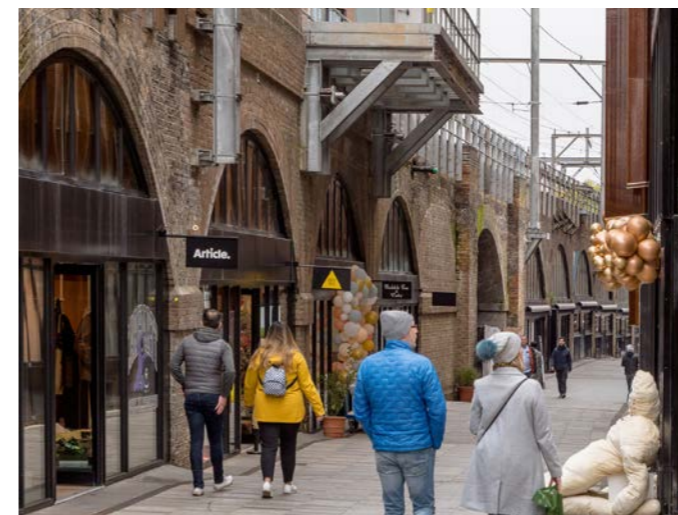
Development along railway arches, Hawley Wharf
