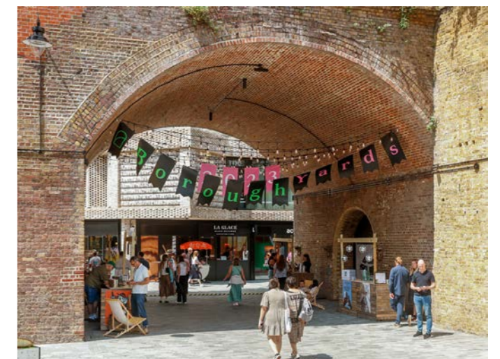
Active railway arches, Borough Yards
