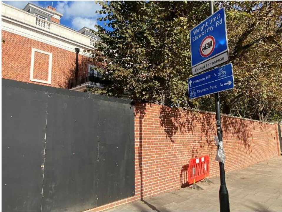
3.4 Dibonded and current temporary hoarding (approximately between August and October 2022)
