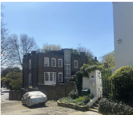
Above: Photo of existing rear elevation.
