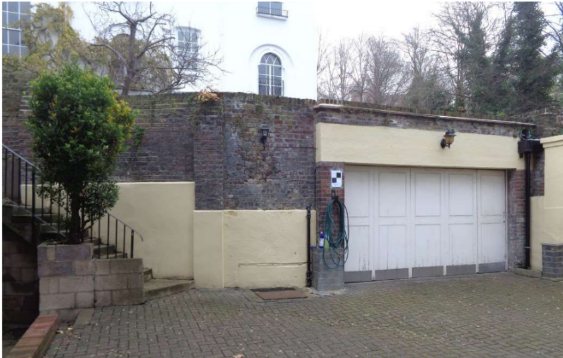
Above: Photograph of the garage area as seen from 99 Frogna
