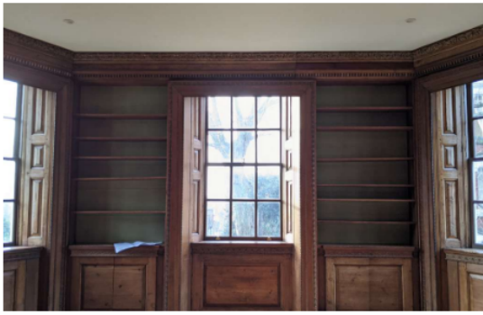
Above: Central room, looking south
