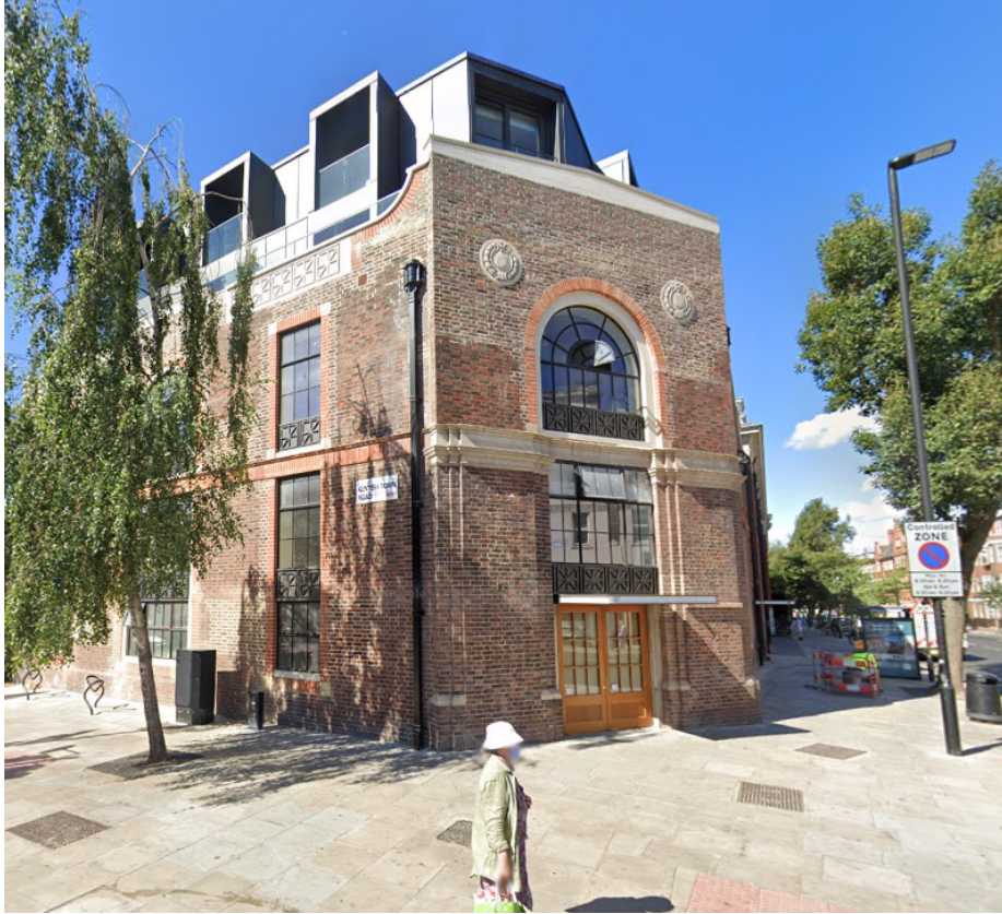
Image 1 – street view of application site
