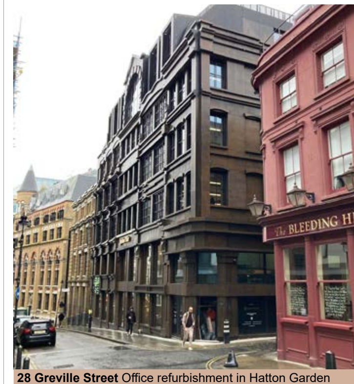
28 Greville Street Office refurbishment in Hatton Garden
