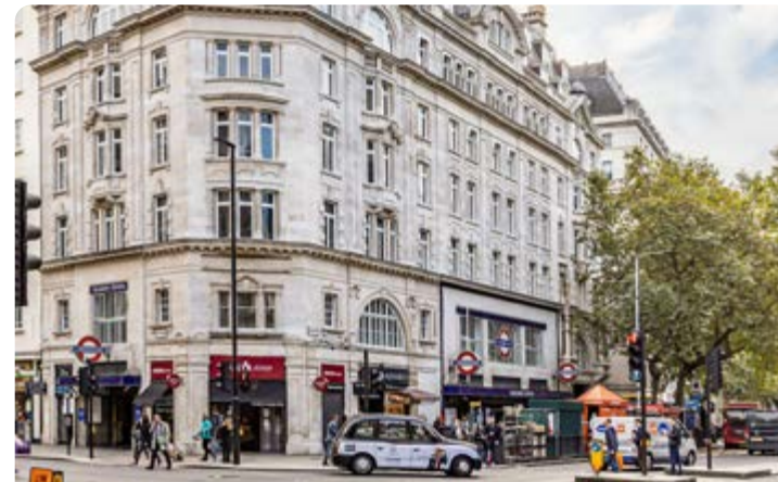
Holborn tube station from the junction (from LDA report)
