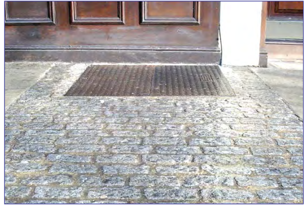
Granite setts laid in front of a cellar flap
