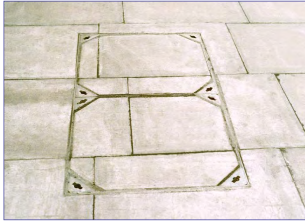
Inset inspection cover showing careful alignment of paving bonds
