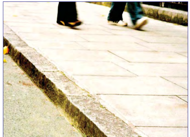
Boulevard paving laid with 150mm staggered bond
