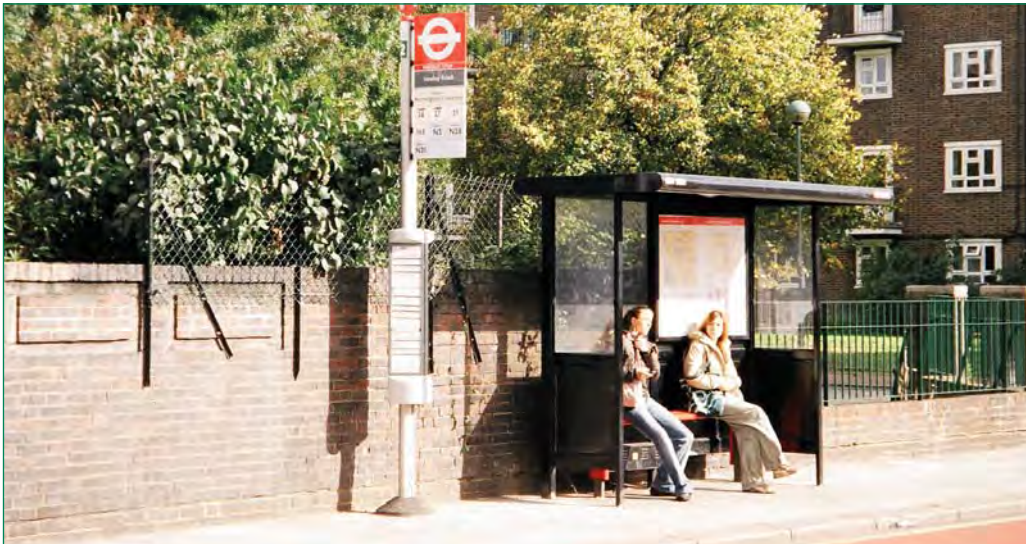
Bus shelter neatly positioned at back of footway
