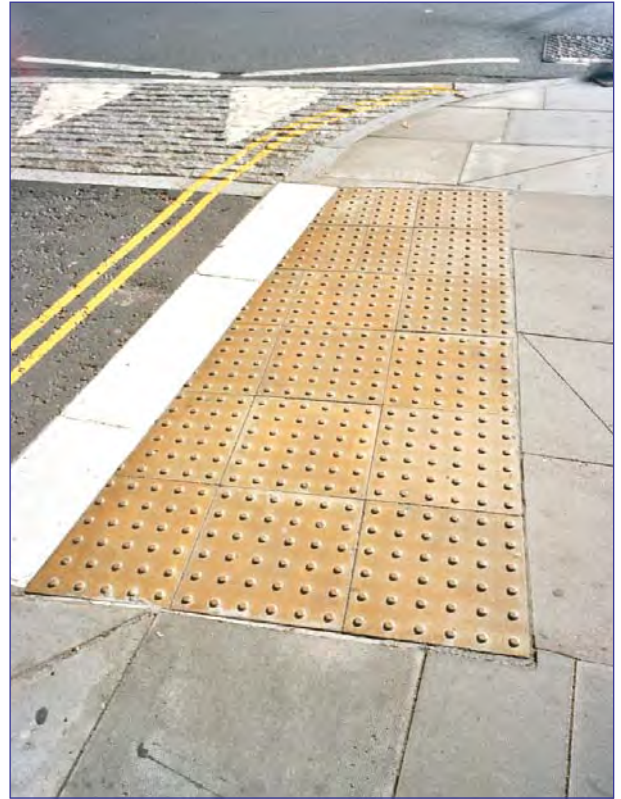
Buff tactile paving at an uncontrolled crossing, on a raised entry treatment
