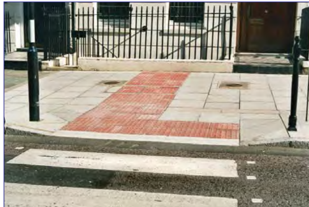
Red tactile paving with stem at controlled crossing
