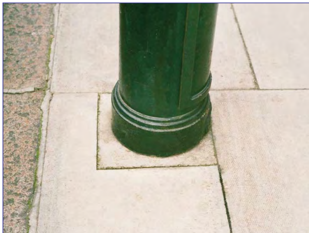
Careful attention to cutting slabs around street furniture
