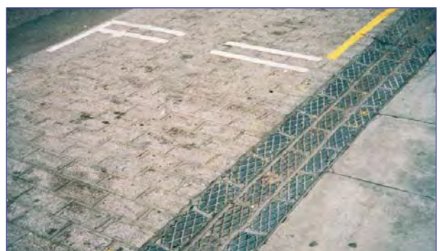
Setts in level loading bay in Chalk Farm Road
