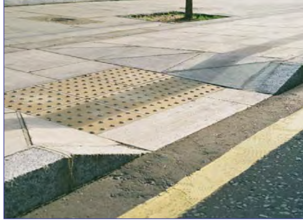
Details of dropped kerbing in John St
