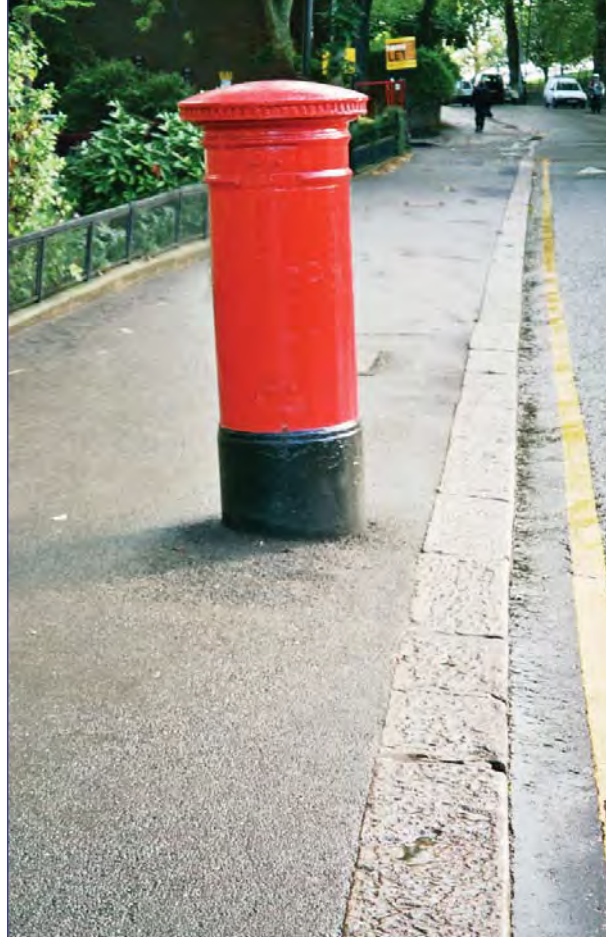
New bituminous footway on Regent's Park Road
