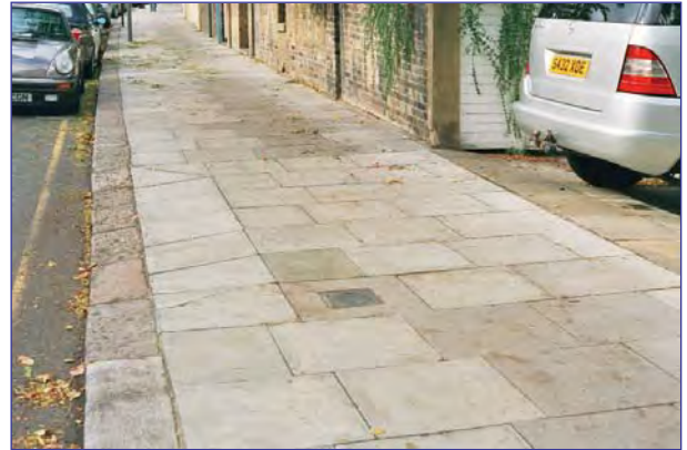
Level footway maintained at crossover with continuous paving
