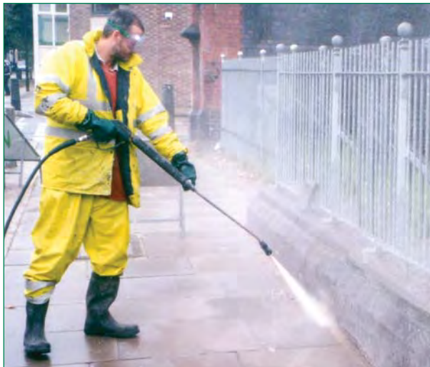
High pressure washing of Boulevard footway
