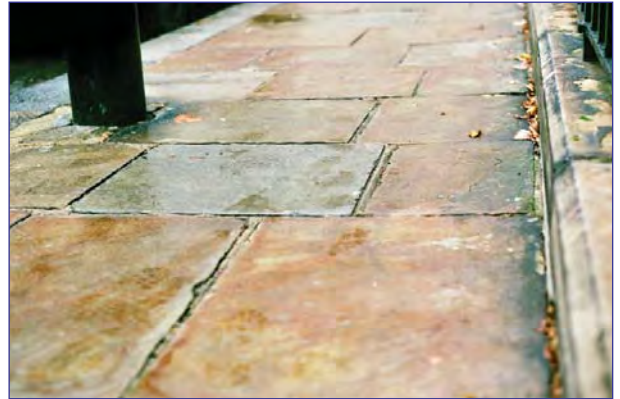
Old York stone re-laid with flush pointing
