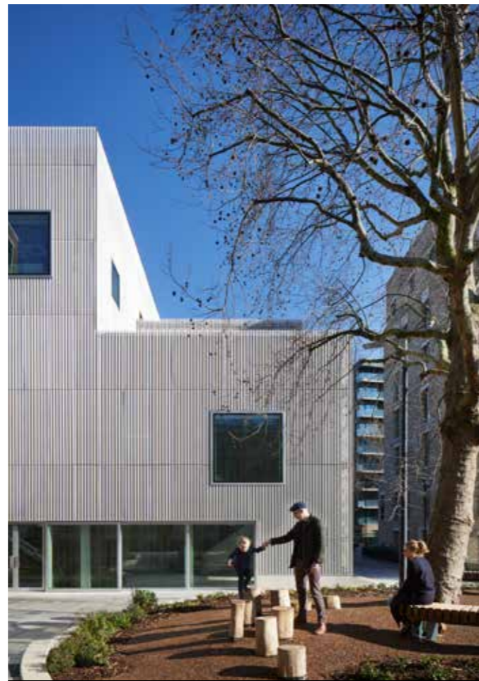
Energy hub with community spaces, Southwark by Morris+Company
