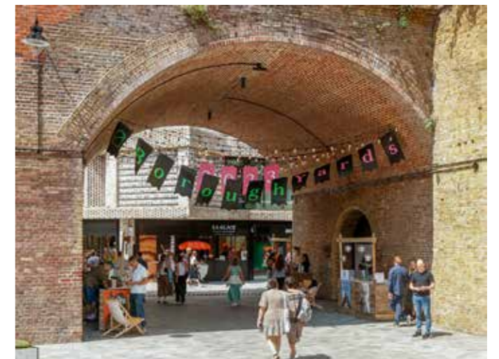
Active railway arches Borough Yards
