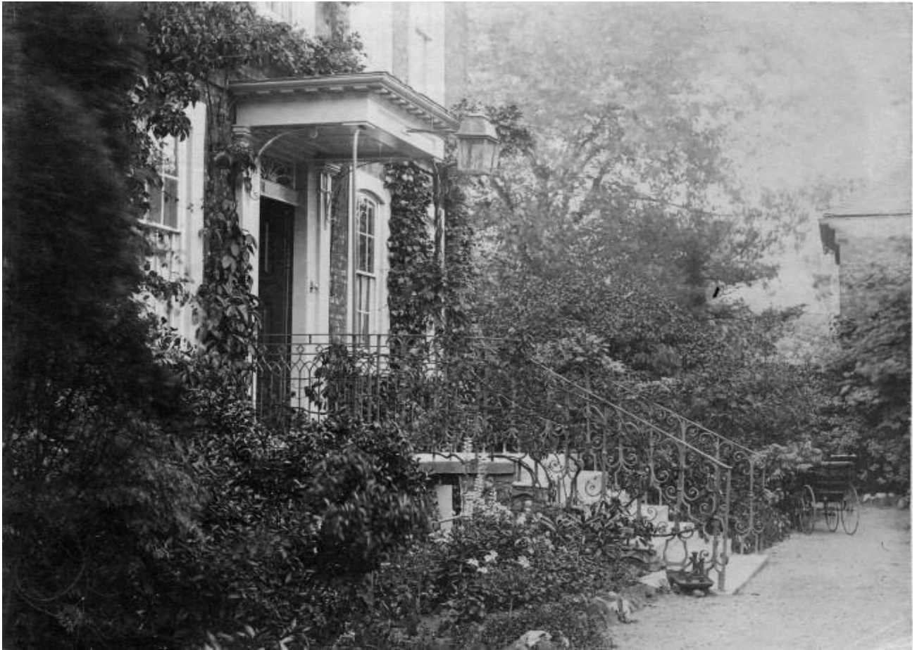
c1884-97 Burgh House front steps
