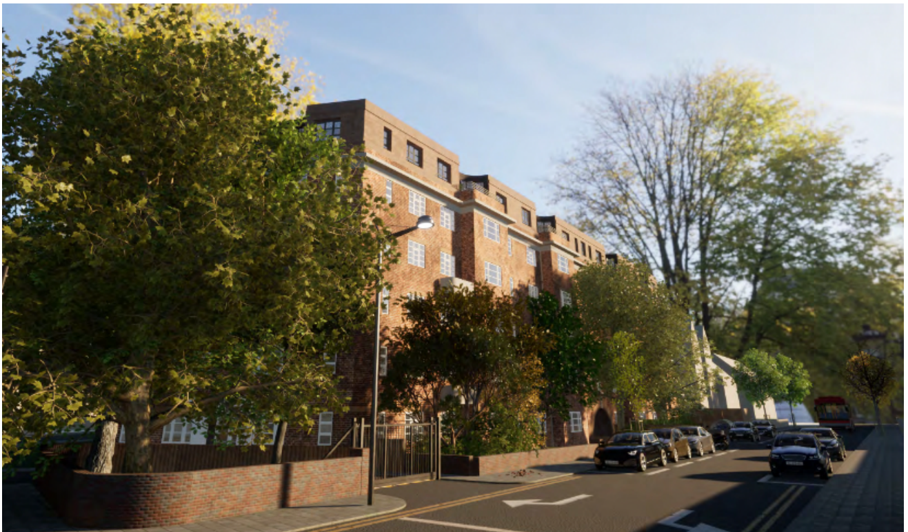
10. 3D visual showing proposed roof extension from intersection of West End Lane and Cleve Road.
