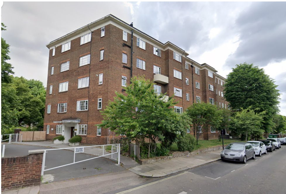
2. Picture of south elevation of building facing Cleve Road as existing
