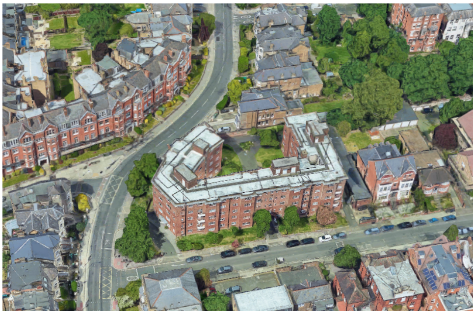
Figure 1 – The existing site
