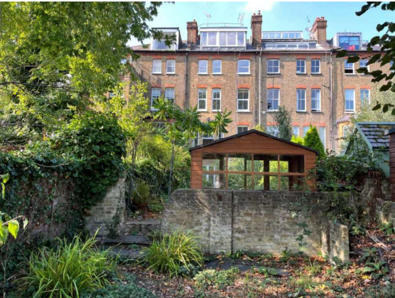
Fig 5. (Above) Existing outbuilding, view from rear
