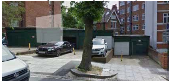
Photo 20: Frognal Lane Garages, Streetscape
