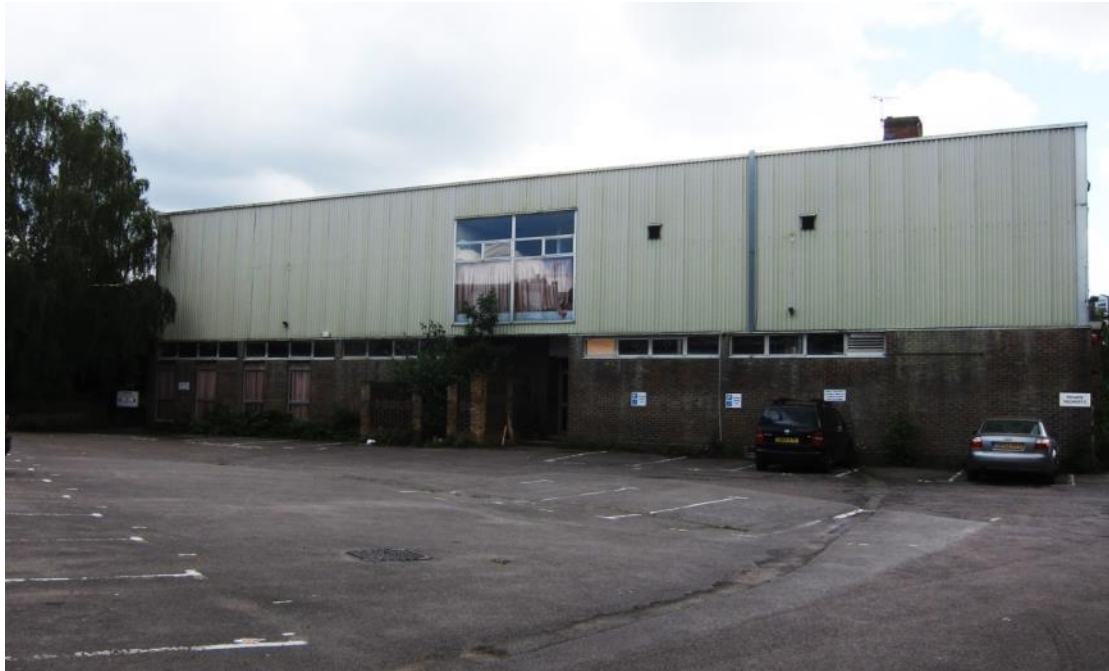
Mansfield Bowling Club (before demolition)
