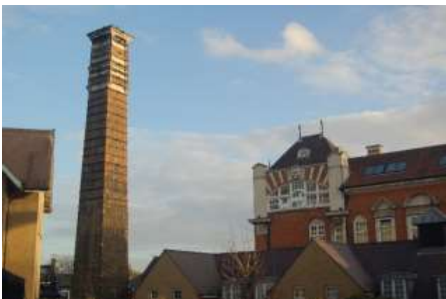
Former New End Hospital Chimney above adds variety to the landscape while Natwest Bank skyline, with oversized dormers, below, destroys the scale of the street
