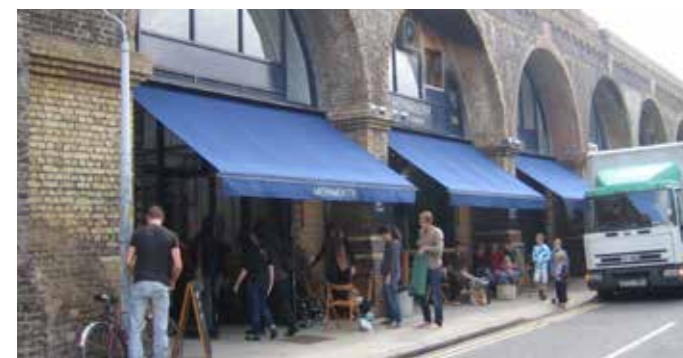
Railway arches providing activity
