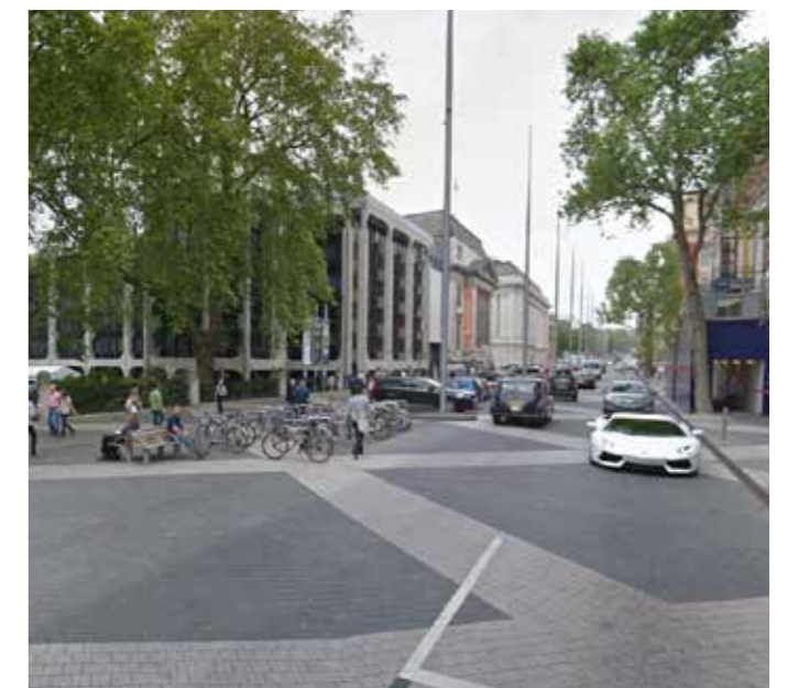
Attractive shared surface on exhibition road in Kensington and Chelsea by Dixon Jones
