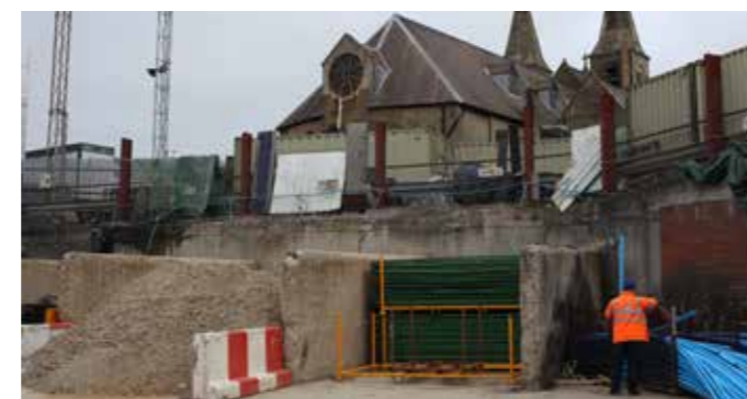
Significant level changes
