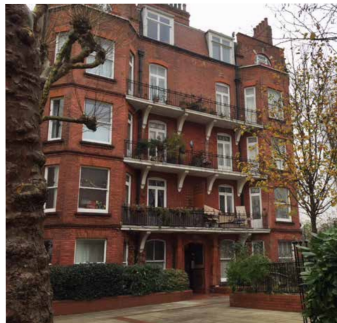
Mansion blocks, Lissenden Gardens
