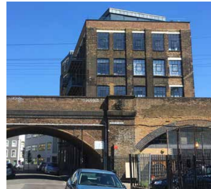
Warehouse buildings and railway arches, Wilkin St Mews
