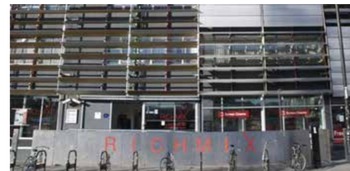
Community and cultural building, Rich Mix
