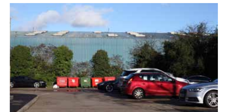
Poor quality buildings and public realm
