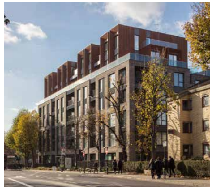
Camden Courtyards by Sheppard Robson Architects
