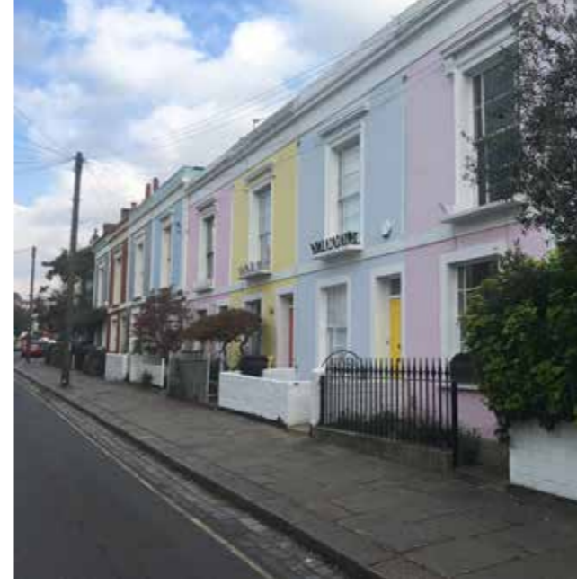
Kentish Town Conservation Area
