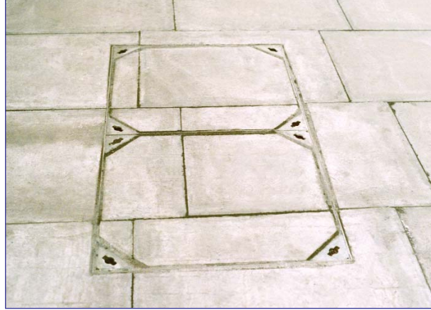
Inset inspection cover showing careful alignment of paving bonds
