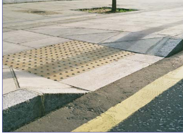
Details of dropped kerbing in John St
