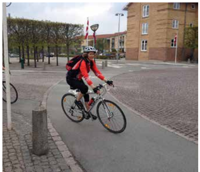
Type 3 - Copenhagen (Furesø): small roundabout with an-ular cycle lane
