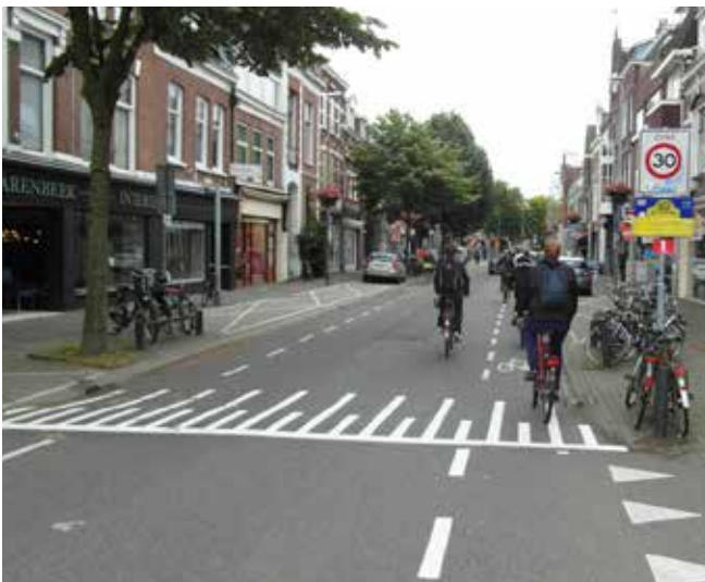
Utrecht - lower speed limit on a high street where space restrictions preclude physically separated tracks
