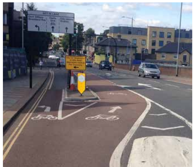
Cambridge: left turning & ahead cycles split approaching the zone where left-turning general traffic crosses
