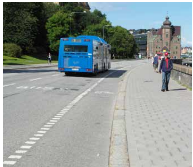
Cycle lane inside fully-specified bus lane - Stockholm
