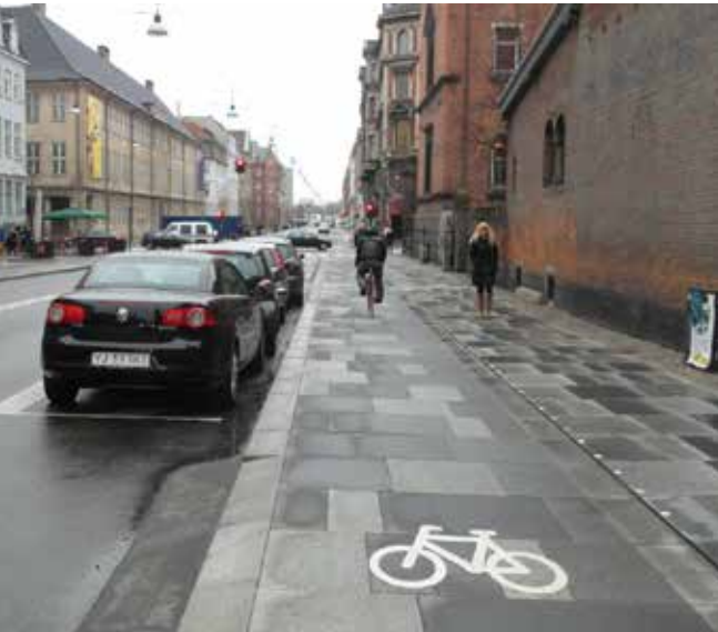
Copenhagen: same materials used for cycle and foot paths on Vester Voldgade; small step and metal studs separate
