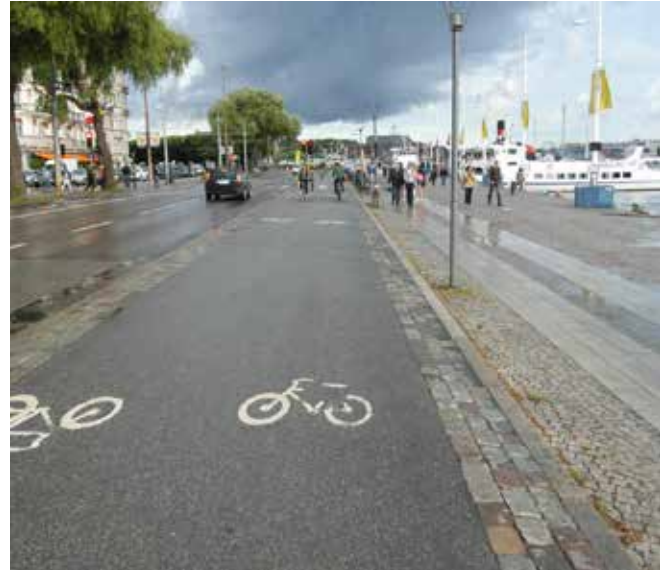
Bi-directional tracks are commoner where there is one-sided frontage (Stockholm waterfront to right)
