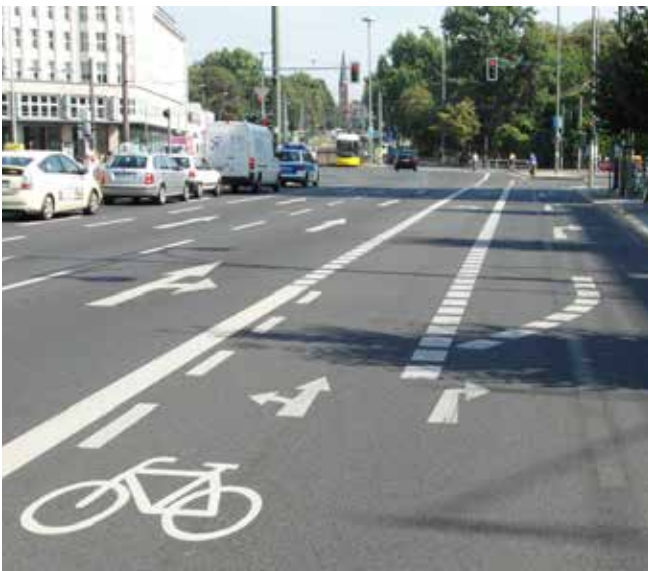
Berlin - ahead lane for cycles with mixed nearside turning lane.
