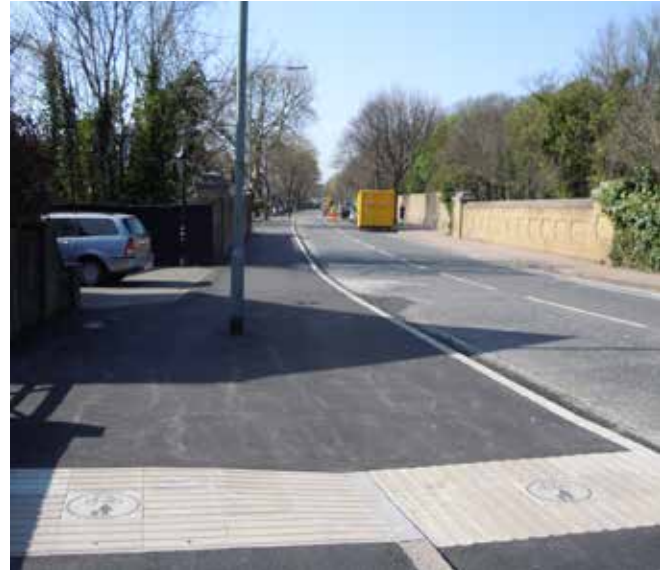
Brighton & Hove: where the Old Shoreham Road narrows, separate cycle & foot paths merge into a wide shared path
