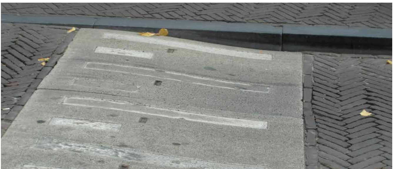
Amsterdam - sinusoidal ramp profiles make for a very smooth ride
