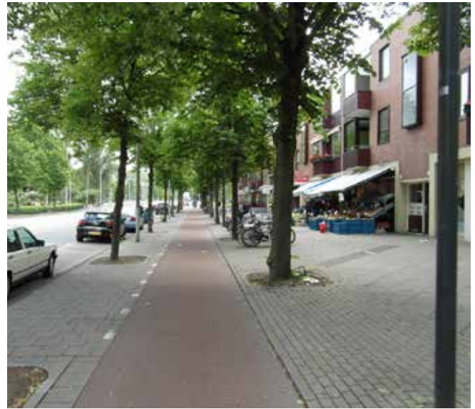
A fairly typical arrangement in Amsterdam, outside the historic centre: carriageway; parking; cycle track; footway
