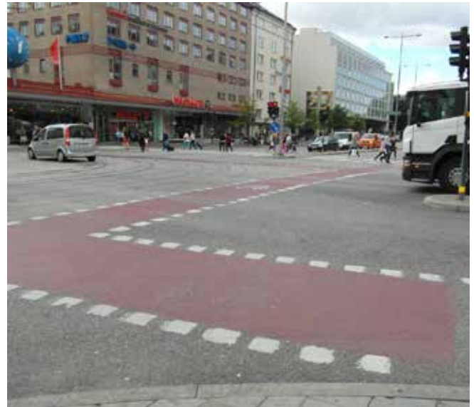
Stockholm - bounded colour used to denote the cycle lanes through a busy crossroads
