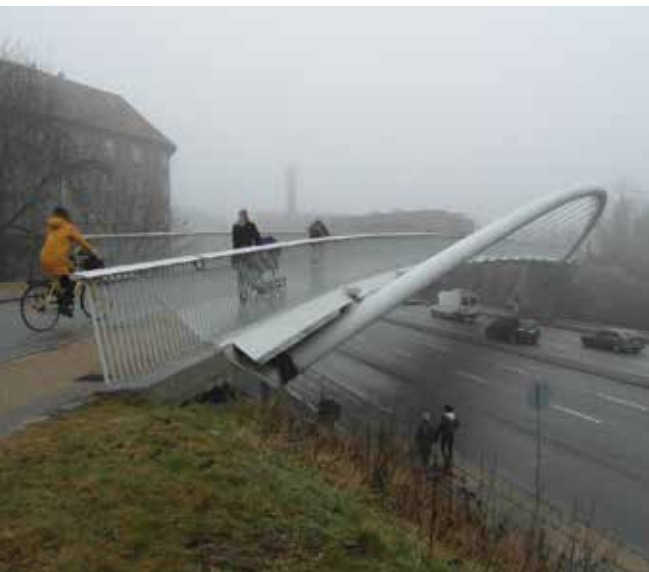
Copenhagen - a purpose-built pedestrian-cycle bridge over a major highway.
