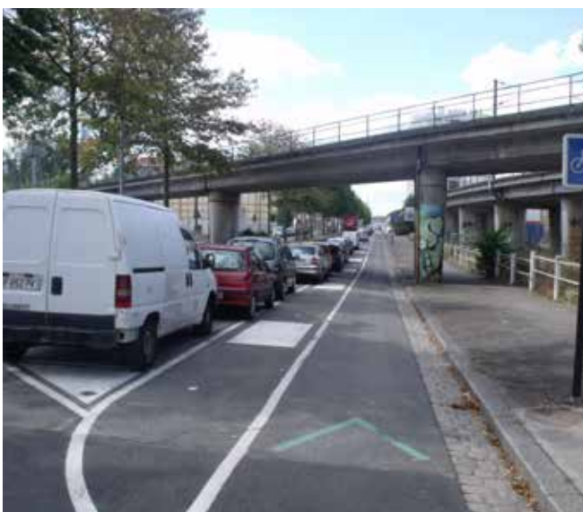
Wide buffer strip with offside parking: Nantes
