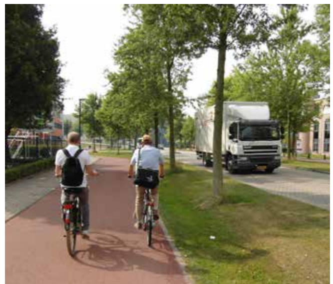
In Houten, near Utrecht, this cycle track is separated from the carriageway by a generous verge and trees
