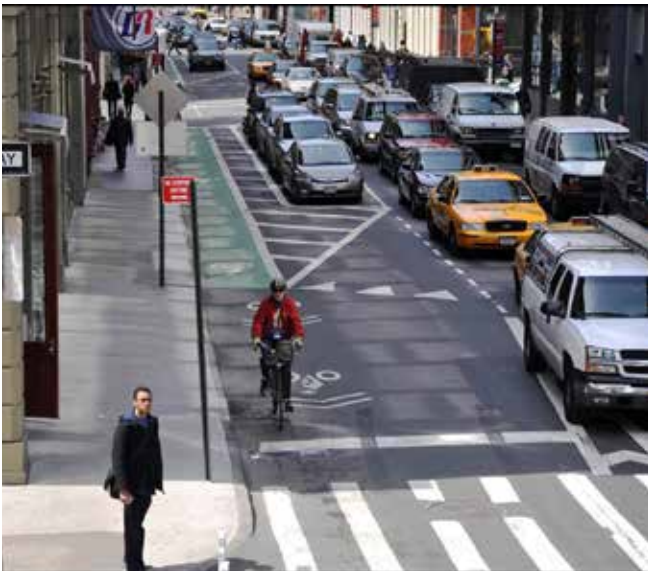
New York - 'Mixing zone' where green lane colouring is cut short to show that cyclists do not have absolute priority
