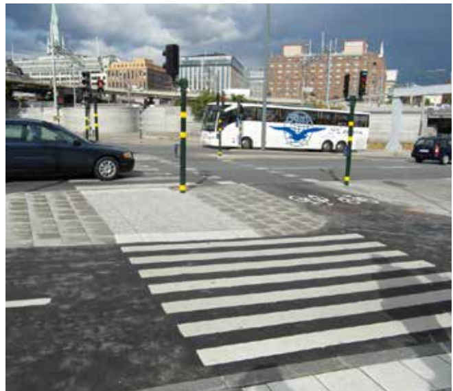
Signalised, mid-link, parallel pedestrian and cycle crossing in Stockholm
