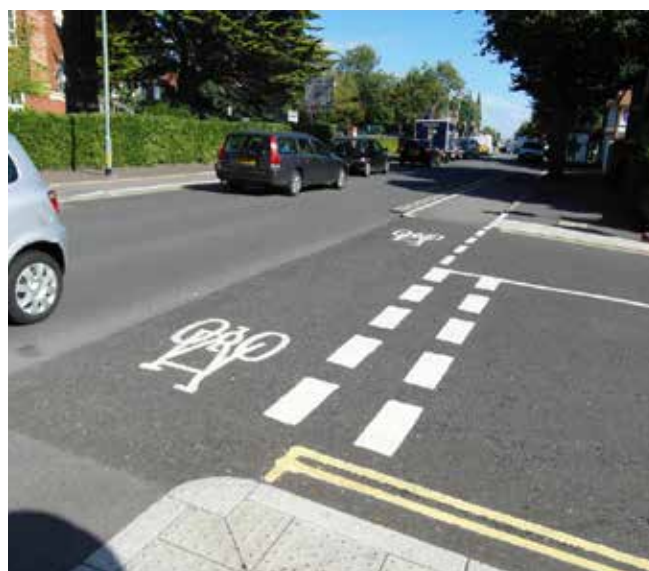
Brighton & Hove - typical treatment on the Old Shoreham Road as the cycle track crosses a minor side street
