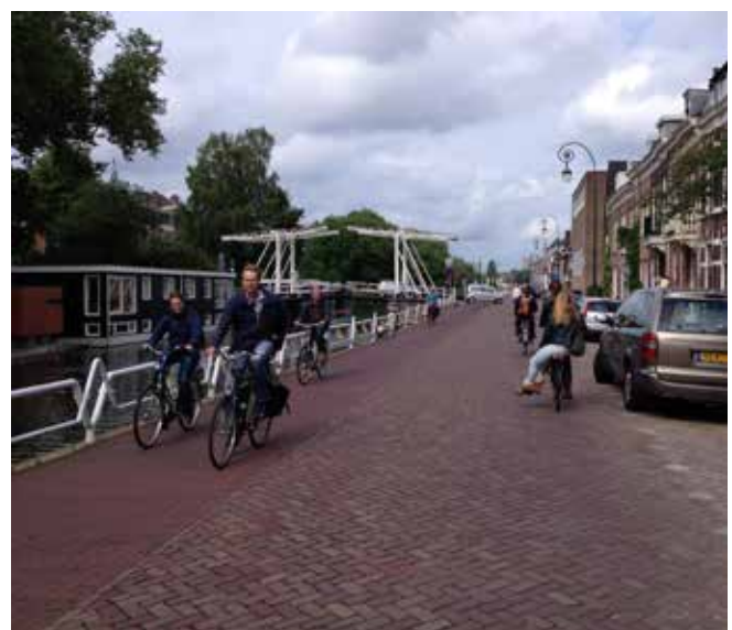
Utrecht - contra-flow on the grand scale: a one-way street with one-way cycle track in the other direction alongside
