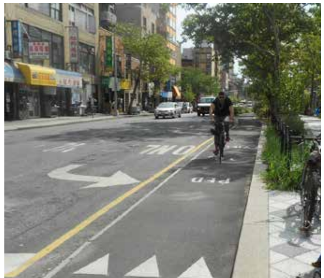
New York - stepped track as part of public realm scheme
