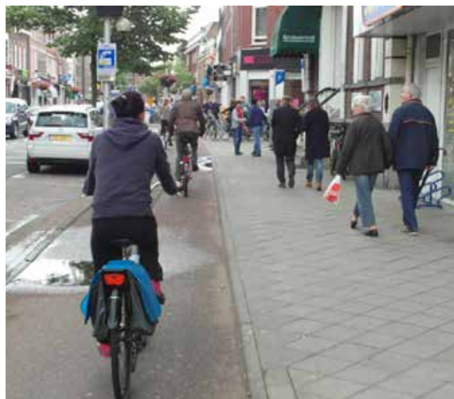
Amsterdam: distinct materials, as well as a step, used to separate adjacent cycle track and footway
