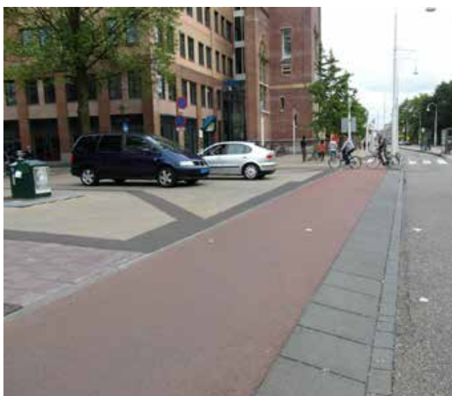
Utrecht - cycle track priority over the side street is emphasised by use of coloured asphalt
