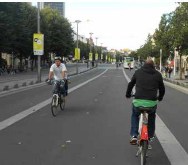
A central, raised bi-directional track between bus lanes on Cours des 50 Otages in Nantes
