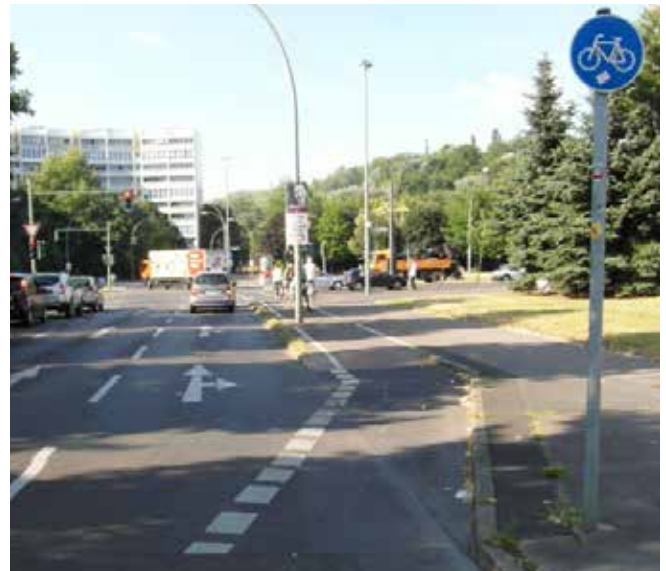
Berlin: transition from an on-carriageway lane to a stepped track on the approach to a signalised junction
