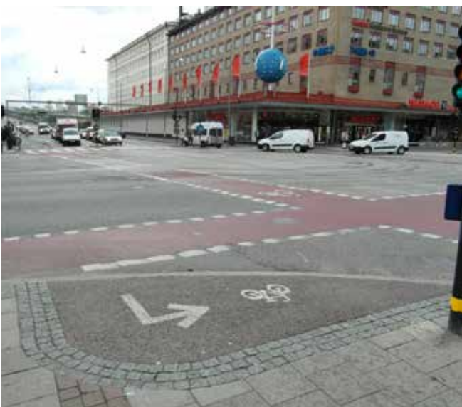
Stockholm - a waiting pocket just off the main carriageway
