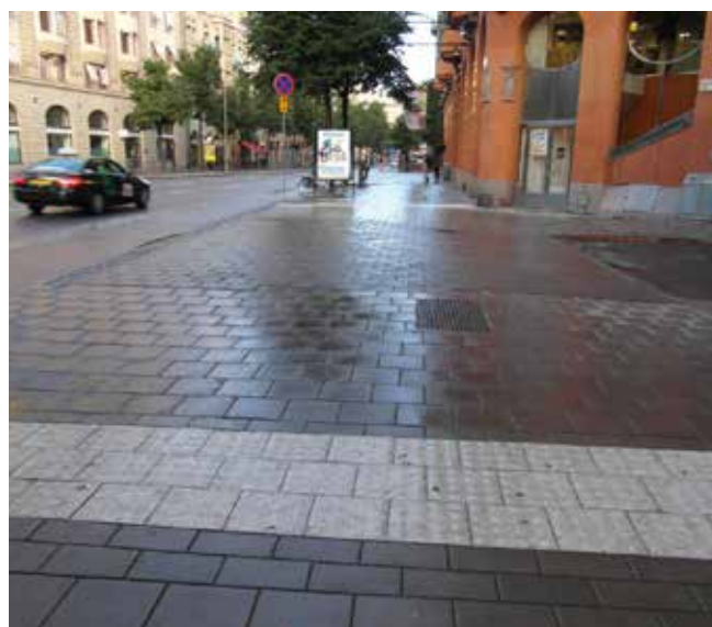
Stockholm - continuous, wide foot/cycle-path across a side street junction
