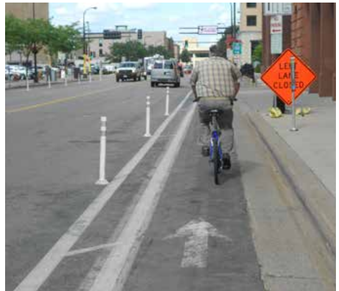
Flexible wands, with painted buffer strip: Minneapolis
