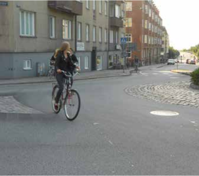
Type 1 - Lund: 'Continental' geometry roundabout with no cycle facilities
