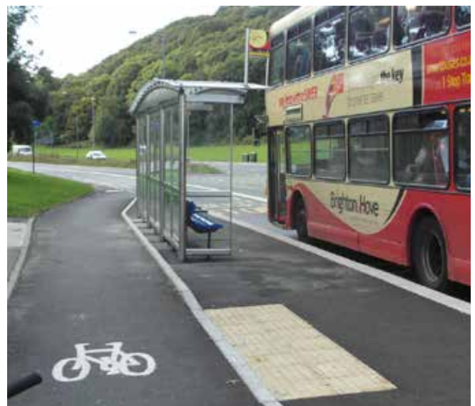
This is the standard bypass layout along most of the Lewes Road cycle track in Brighton & Hove
