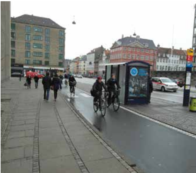
Bus stop bypasses are commonplace in Copenhagen but...
