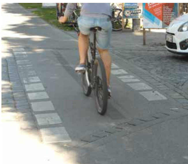
Munich - simple markings and materials help emphasise cycle priority as the track crosses a side street
