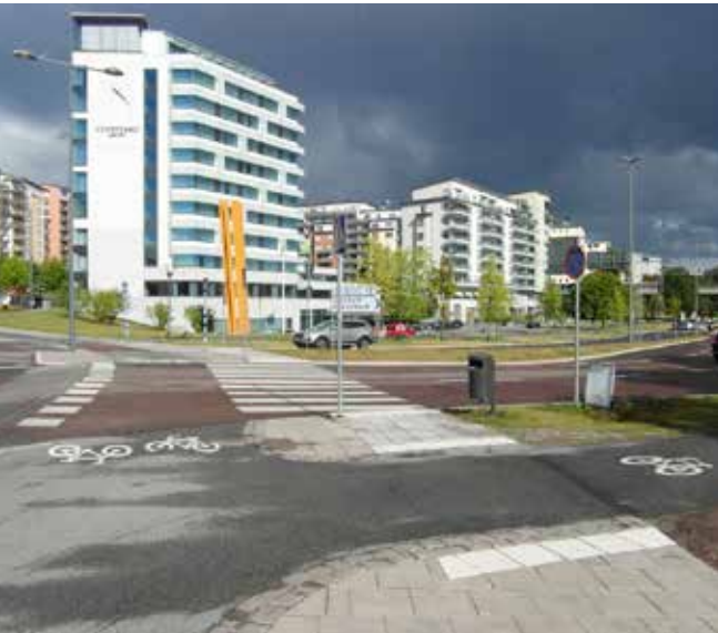
Unsignalled crossing at a roundabout in Stockholm - pedestrians have priority over motor traffic; bicycles do not
