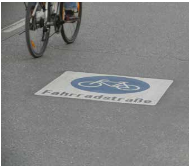
A carriageway marking for a Fahrradstrasse in Munich...
