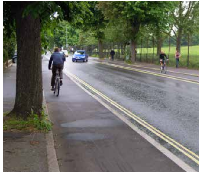
Old Shoreham Road in Brighton & Hove: a 6.1m carriageway with no centre-line between stepped cycle tracks
