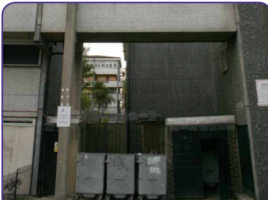
Inactive frontage and external bin stores.
