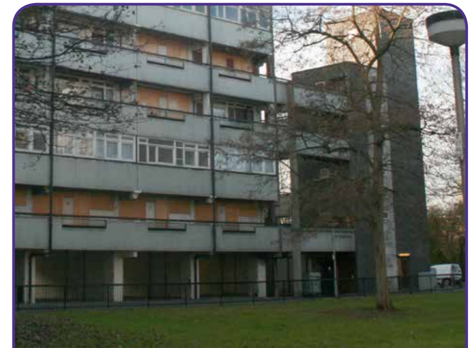
carports at ground floor create inactive frontage and encourage ASB
