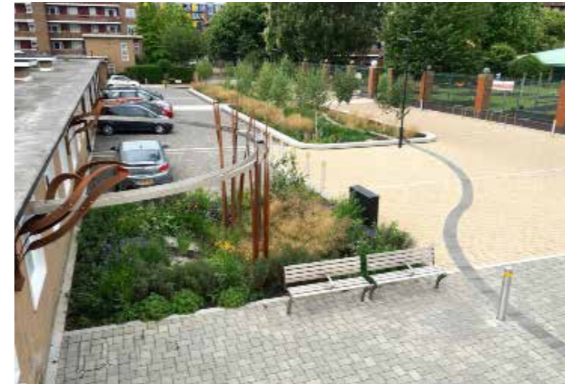
Bridget Joyce Square, London - Parking space turned into a green space with use of SuDS and increased biodiversity
