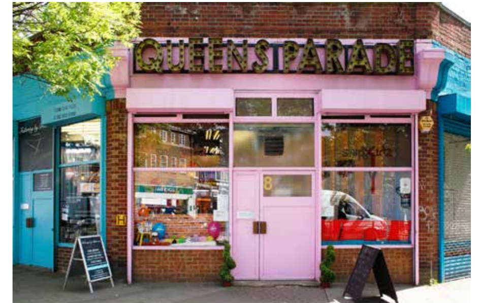
Queens Parade, Willesden Green - Meanwhile use project to provide affordable retail units for the local community on the high street
