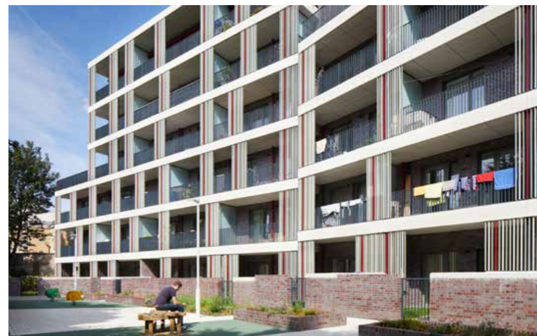
Agar Grove Estate, Camden - council-led net-zero housing development that follows the principles of Passivhaus design, also tackling fuel poverty. Photo Credit: ©Jim Stephenson
