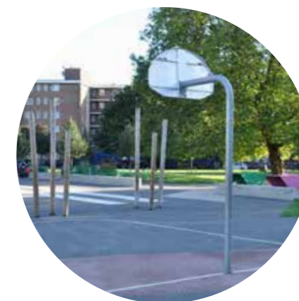
Stonebridge gardens, Hackney - Former MUGA in poor repair replaced with an informal sports area inclusive to a greater range of residents
